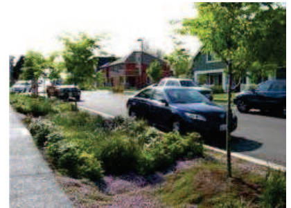
A street swale in Seattle
